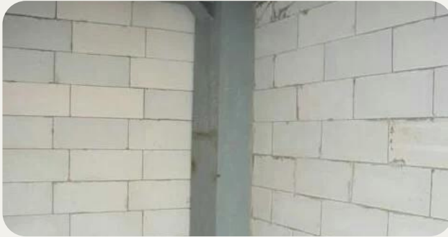
05 ACC BLOCK PLASTER
